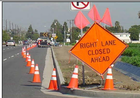
Figure 1: Traffic Control, Lane Closure (typical)
