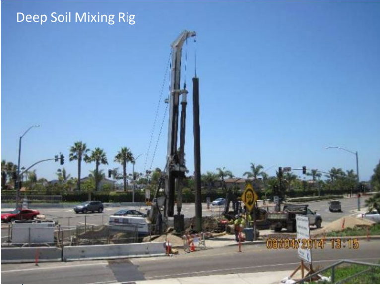
Tri-Axis Auger Mixing Rig
