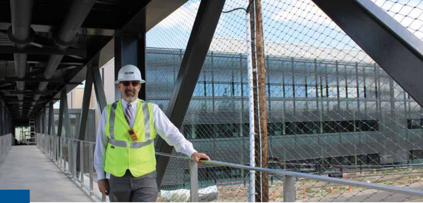
GM Rob Thompson on the new bridge over Ellis connecting the new headquarters to the FV plant.
