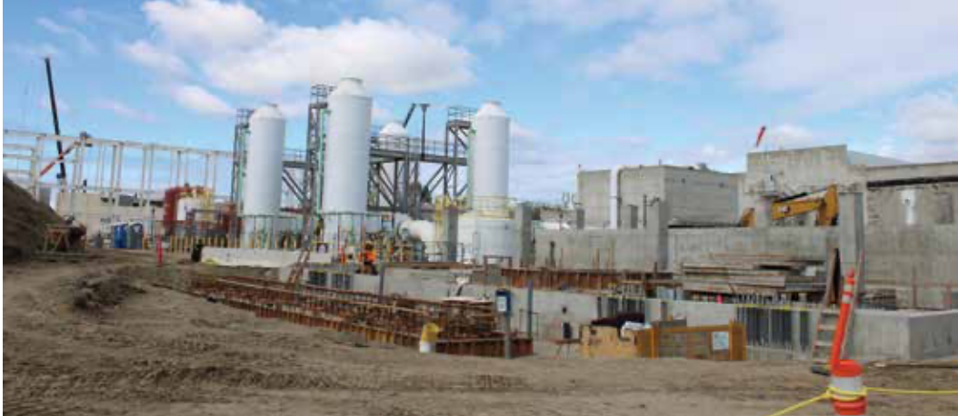
Upgrade of the FV Headworks facility – where the treatment process begins.
